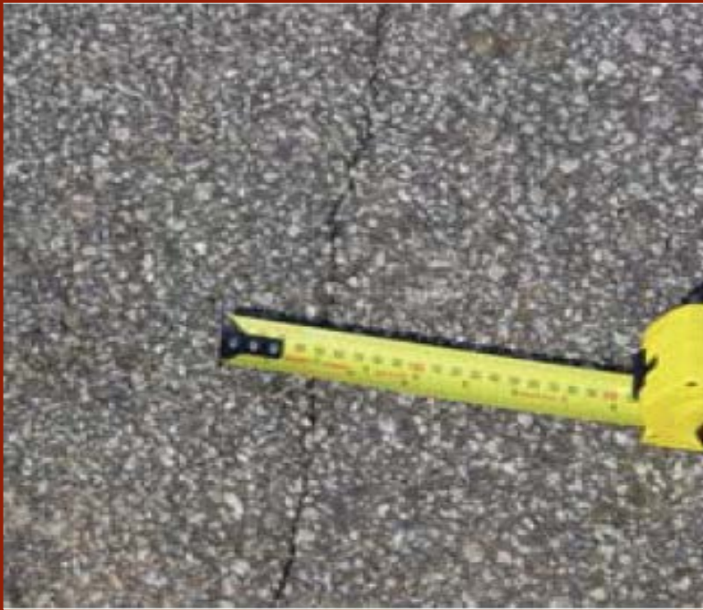
Narrow Cracks
