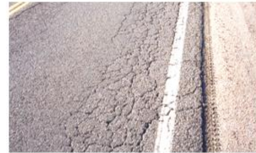
Fatigue Cracking
