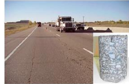
Top-down Cracking
