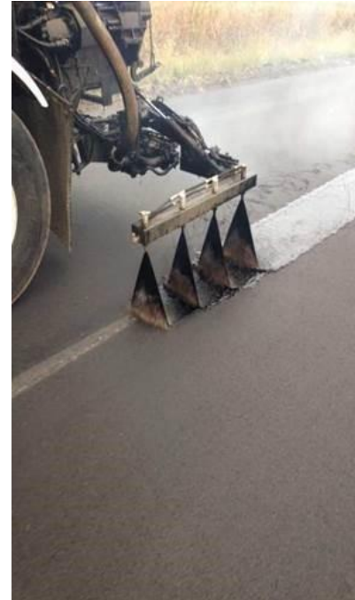
Longitudinal Joint Seal
