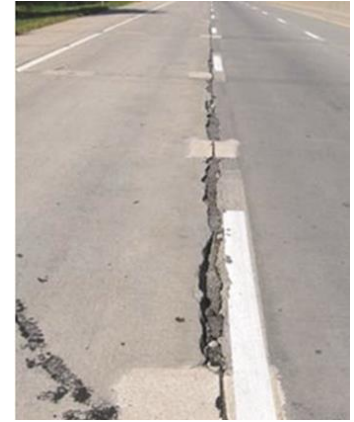
Joint Spalling
