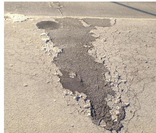
D-Cracking
