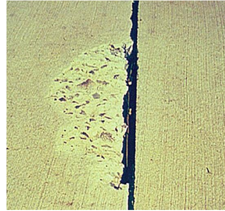
Joint Spalling
