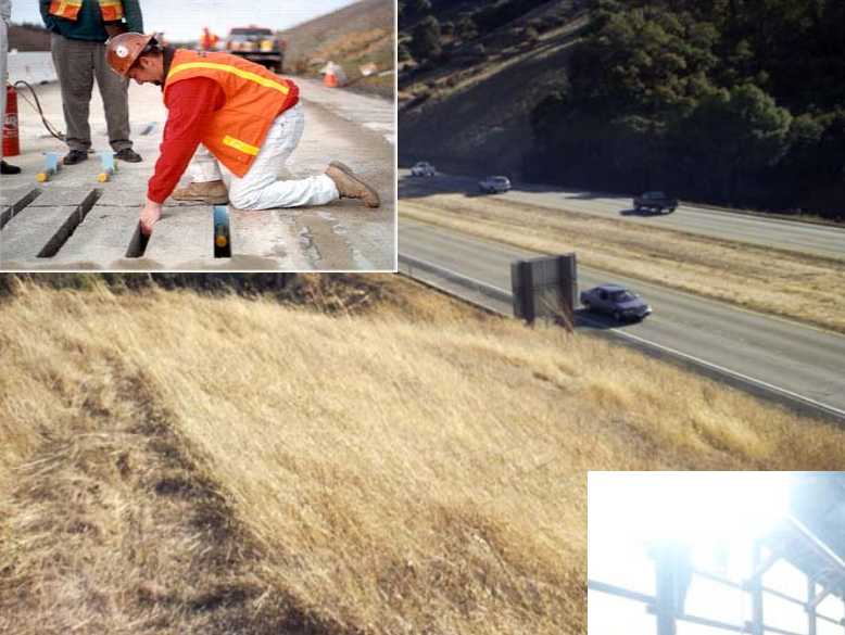
Ukiah, CA Dowel Bar Retrofit
